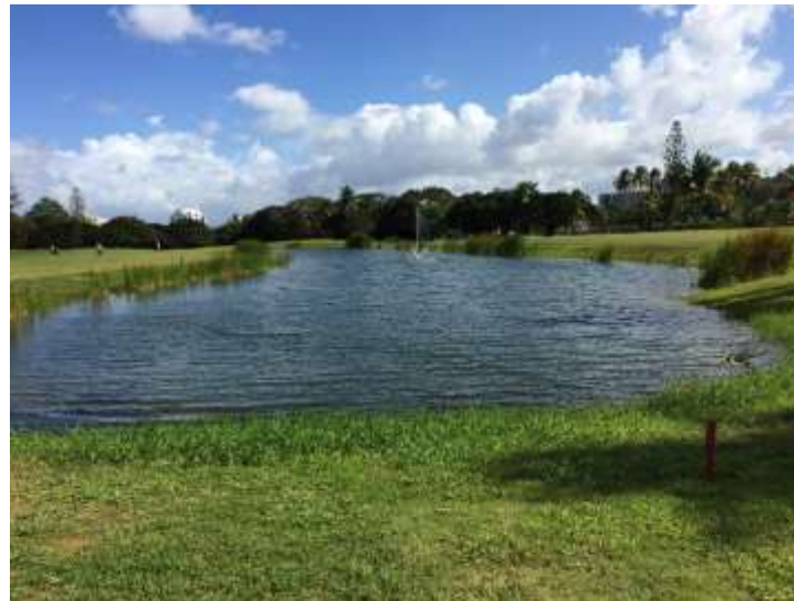
Golf Course Irrigation System, Fort Buchanan, PR ESPC
