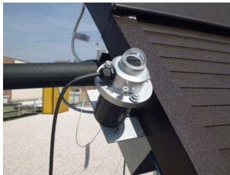
Figure 10 - The monitoring system: pyrometer
