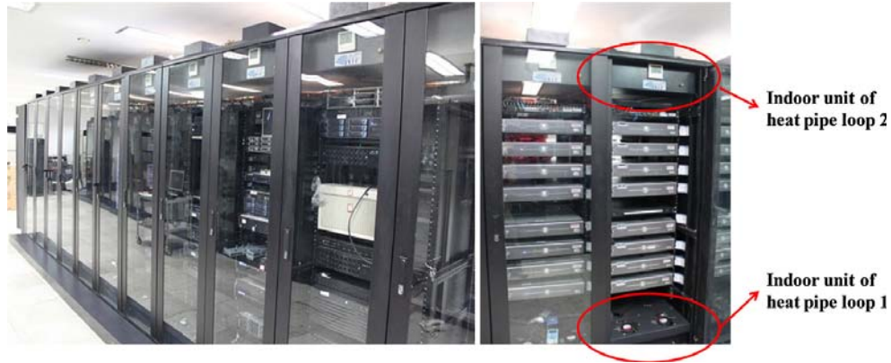
Fig. 3-11. Internally cooled racks using two-stage heat pipe loops.
