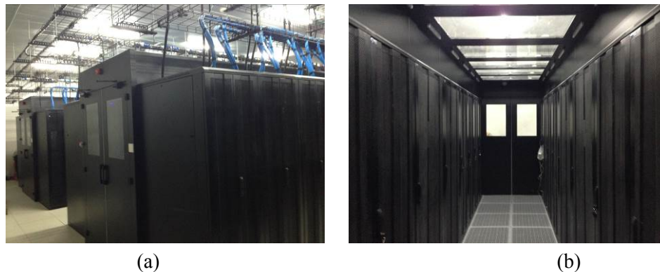
Fig. 3-1 Schematics of classical data center and cold aisle: (a) Schematic of a data center; and (b) Closed cold aisle.
