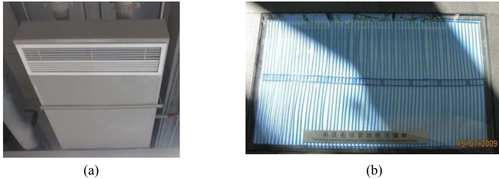
Fig. 0-6 Indoor terminal devices: (a) dry fan coil unit; (b) capillary radiant panel.
