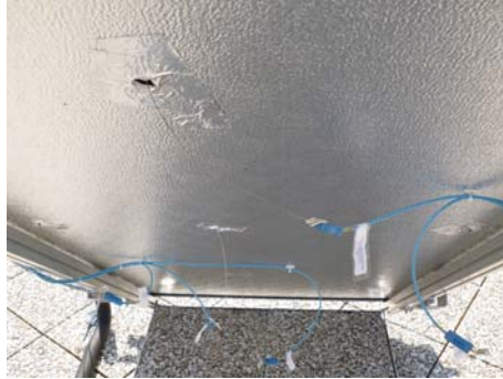
Figure 9 - The monitoring system: thermocouples
