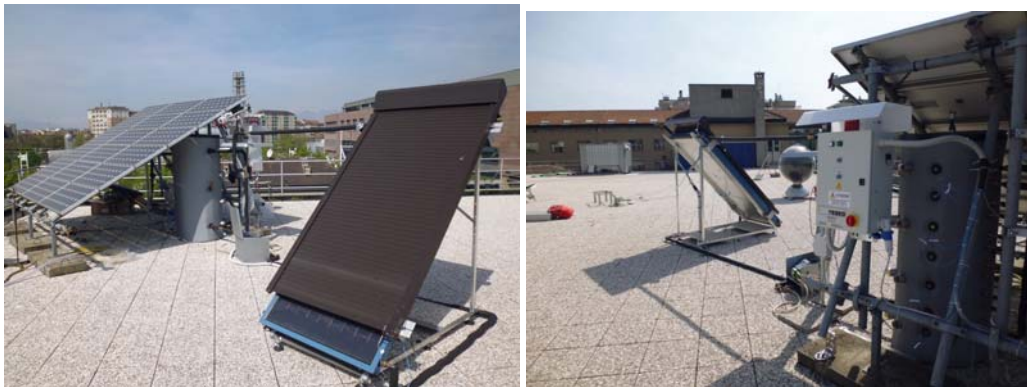
Figure 5 - The real-scale prototype: general view and details of the storage tank and the electronic control unit.
