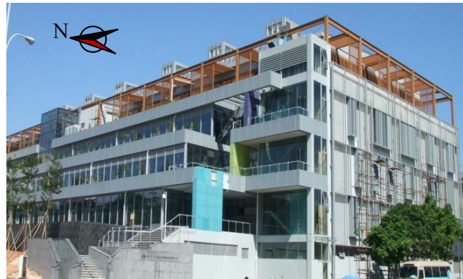
Fig. 0-1 The tested office building in Shenzhen.
