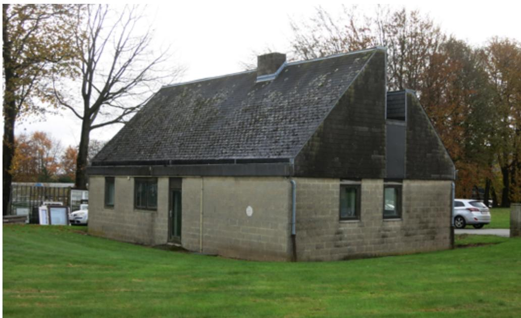
The IDEE house at Limelette, Belgium, a full-scale experimental building that has been used as a test case to develop and evaluate methodologies to characterise the overall heat loss coefficient based on static and dynamic measurement campaigns.
