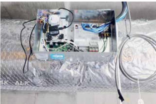
A variable air volume unit being monitored for signal exchanges and the angle of the opening control valve.
