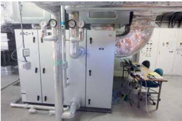
An air handling unit being monitored for fan speed, airflow rate and energy use.
