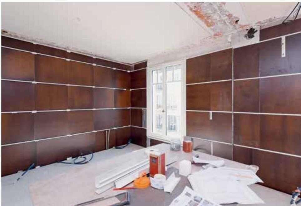
Indoor renovation with vacuum insulation panels finished with a protective layer.
