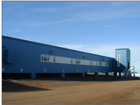
Figure 5-5. Examples of elevated structures on permafrost. Upper photo: An image of downtown Utqiagvik, Alaska where single-story and multi-story buildings, as well as all utilidors, are constructed above ground. Lower left: a large facility at Prudhoe Bay, Alaska. Lower right: a single-story structure at Thule, Greenland. Photos by Kevin Bjella, CRREL.
