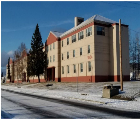
Image 8-1. Building 2 Concrete Wall/Steel Roof
