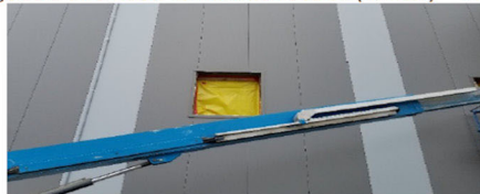
Image 11-4 IMP Louver Termination Sealed
