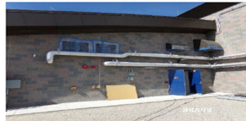
Image 11-5 CMU Louver Wall Termination Sealed
