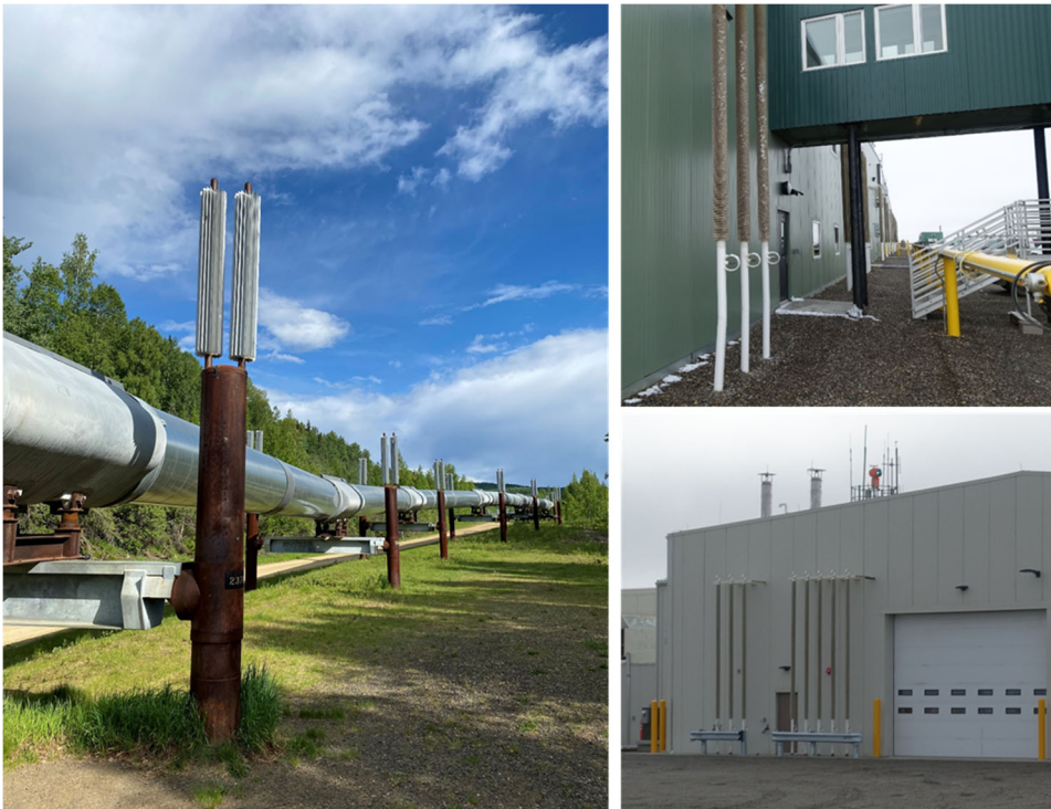
Figure 5-7. Images of thermosyphon installations. Left: on the Trans-Alaska Pipeline near Fairbanks, Alaska. Upper and lower right: along foundation edges of structures in Prudhoe Bay, Alaska. Images by T. Douglas, CRREL.
