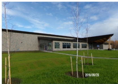
Image 5-1. Bldg. 27 CMU Wall & Metal Roof
