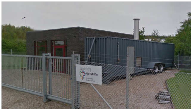
Figure 7-11. Portable emergency boiler in the Sønderborg district heating system.
