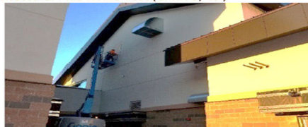
Image 11-3 EIFS Louver Wall Termination Sealed (Winter)
