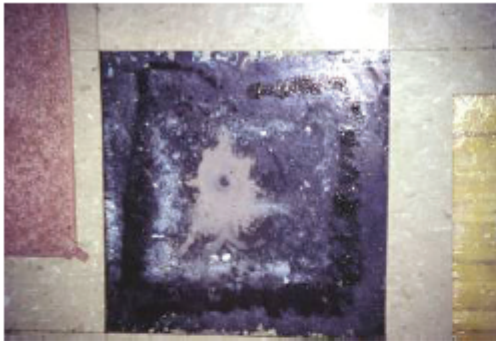
Figure 1-13 Tile adhesive that failed to cure because of water in the concrete and high pH. The tile can be removed by hand. The floor is a concrete slab-on-grade. The water visible in the photo evaporates into the room after several minutes. Its source may be liquid water wicking up from the sub-slab fill or water vapor migrating through the slab.
