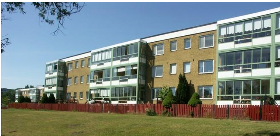
Figure 2. A 3 storey building in Hagalund housing cooperative.
