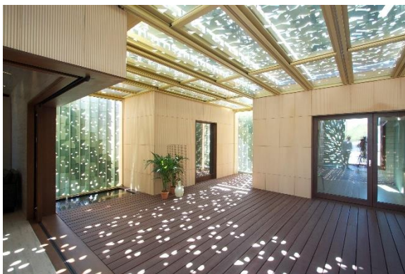
Figure 31: Exterior buffer conservatory at the 2012 AND house, with advanced functionality for the building ventilation concept. Source: SDE, Flickr, Jose Luis Castillo [sde flickr doc]
