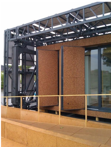
Figure 84: Solar system built over a dominant substructure on the SDE 2012 CEM NEM house (FAU). Source: University Wuppertal: Karsten Voss
