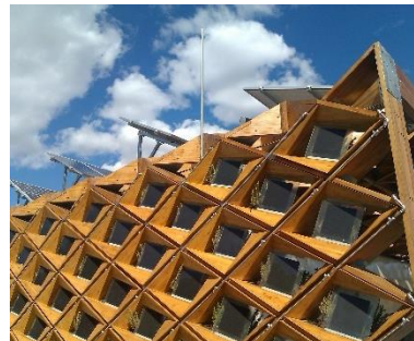
Figure 27: Fixed shading with integrated PV application and planting at the house of the team TJU at SDE 2012. Source: K. Voss, University Wuppertal
