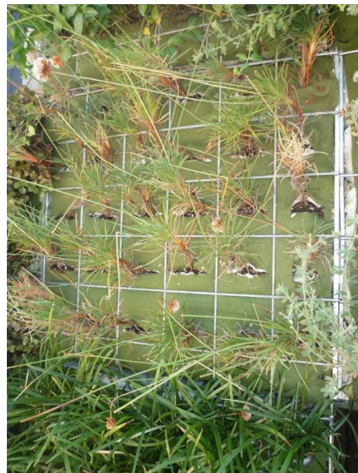
Figure 127: Planted wall to increase humidity in the dry summer climate in Madrid, SDE 2010 without active air conditioning. Source: University Wuppertal
