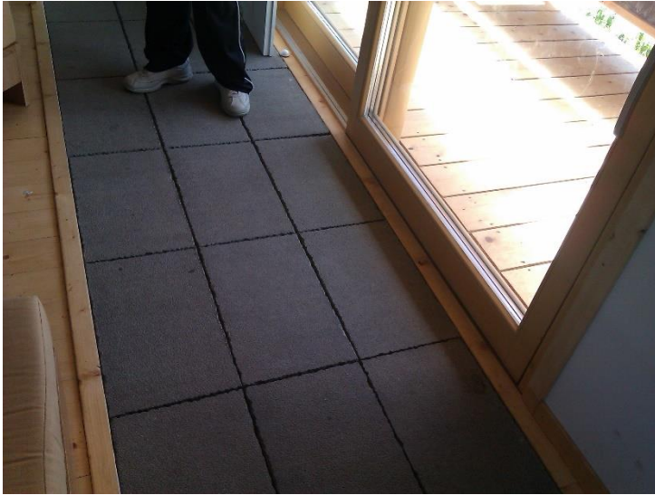
Figure 72: The PRISPA Team at SDE 2012 place thermal mass with concrete floor plates exactly in locations where the sun hits the floor. Source: University Wuppertal, Karsten Voss
