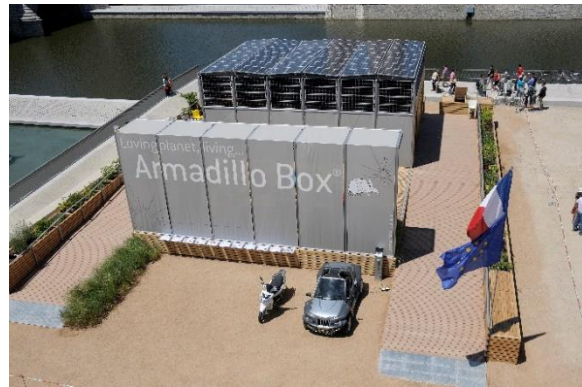
Figure 97: The Armadillo Box created by the French team (GRE) at SDE 2010 also made wide-scale use of photovoltaic systems. The concept used PVT hybrid modules, which covered the roof and the upper section of the building. The solar "hood" on the top of the building is not directly attached to the roof structure and is therefore extremely well ventilated. Source: SDE Flickr, by Javier Alonso Huerta [sde flickr]
