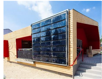
Figure 25: Moveable vertical and external sun protection additionally used for solar power generation presented by the SDE 2014 ROM house. Source: SDE, Flickr, Valeria Anzolin, Jason Flakes [sde flickr doc]
