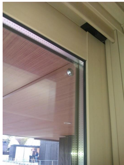
Figure 20: Vacuum glazing at the 2012 Omoenashi House from the Japanese team CUJ. The vacuum double-glazing is combined here with a third pane to a triple glazing unit. Source: University Wuppertal, Karsten Voss
