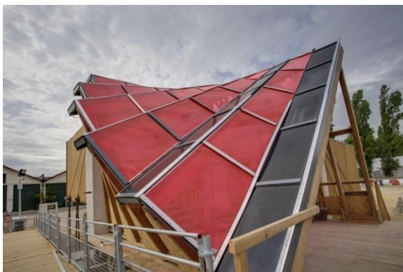
Figure 100: The solar cells in the PAR 2014 house use fluorescent plastic (PMMA) to focus light on solar cells at the edges using total reflection. Source: SDE Flickr, by Valeria Anzolin and Jason Flakes [sde flickr]
