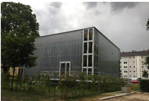
Figure 37: Exterior view of the Cubity house at its most recent location in Frankfurt. Source: University Wuppertal, Victoria Kunz
