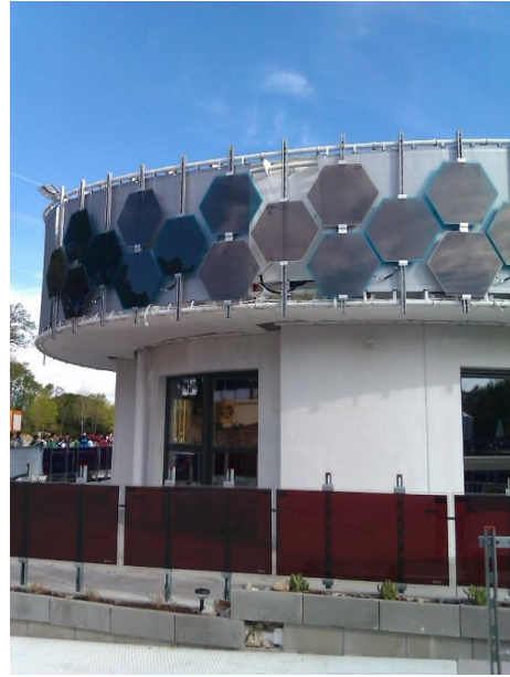
Figure 83: On the SDE 2012 Unizar house (UDZ), solar modules were added to the façade. The hexagonal form of the modules emphasizes the complementary design approach. Source: University Wuppertal, Karsten Voss
