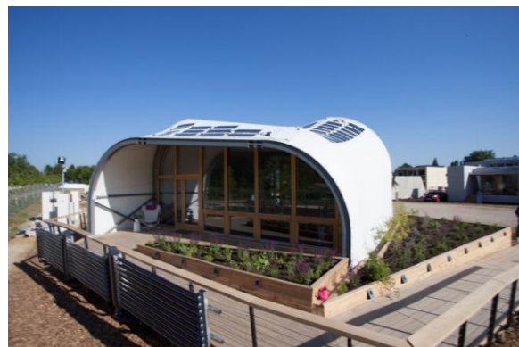
Figure 101: Thin-film modules in the INS 2014 house enable integration into the building envelope, which consists mainly of a membrane. Source: SDE Flickr, by Valeria Anzolin and Jason Flakes [sde flickr]
