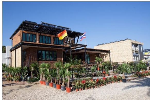
Figure 99: Another example of subtle PV system integration is the OTP 2014 house. Here, modules were only installed on the roof and were almost invisible to the visitors. Source: SDE Flickr, by Valeria Anzolin and Jason Flakes [sde flickr]
