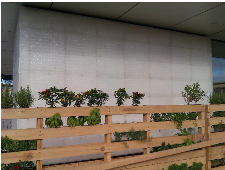
Figure 59: Recycled CDs as external cladding at the 2012 RWT house. Source: University Wuppertal, Karsten Voss
