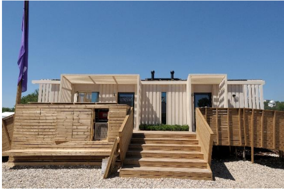
Figure 61: Wooden outside cladding at the SDE 2010 HUT house. Source: SDE, Flickr, Flakes [sde flickr doc]
