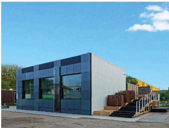
Figure 80: The MOR house (DEF) at SDE 2019 presents a module for high-rise renovation. The façade cladding comprises matt photovoltaic modules which match the colour of the windows by a ceramic ink on the surface. Source: TU Delft, Project Drawings
