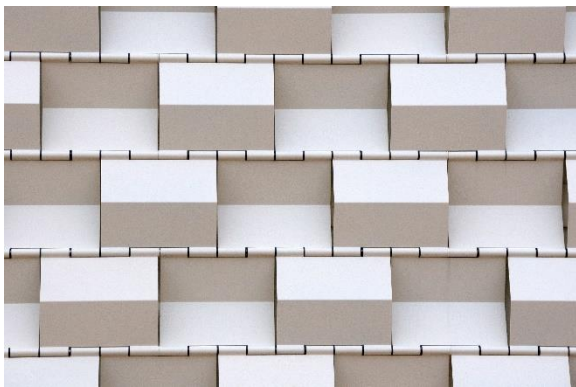
Figure 63: Metal outside cladding on the ventilated façade of the SDE 2010 ROS house. Source: SDE, Flickr [sde flickr doc]
