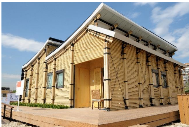
Figure 54: The SDE 2010 TUS house demonstrates the use of bamboo for load bearing as well as cladding. Source: SDE, Flickr [sde flickr doc]
