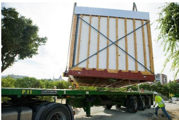
Figure 51: Arrival of one of the modules of the 2012 AND house at the event site. Source: SDE, Flickr [sde flickr doc]
