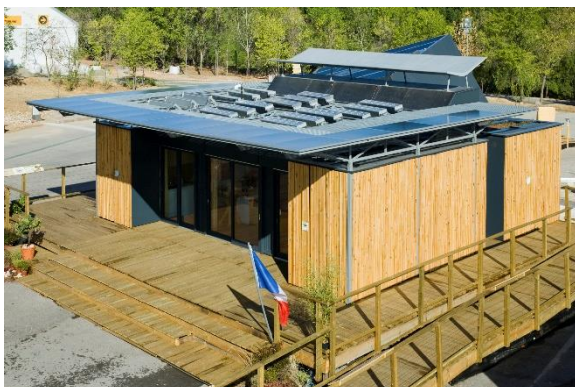
Figure 41: Roof construction with a Venturi wind catcher on the SDE 2012 Symbiosis house (ABC). Source: SDE, Flickr [sde flickr doc]
