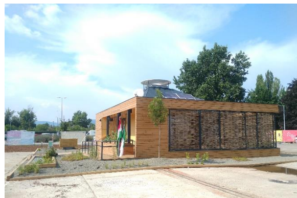
Figure 42: Roof construction of the SDE 2019 MIH house to use the Venturi- effect in addition to a solar chimney for passive ventilation. Source: University Wuppertal, Karsten Voss
