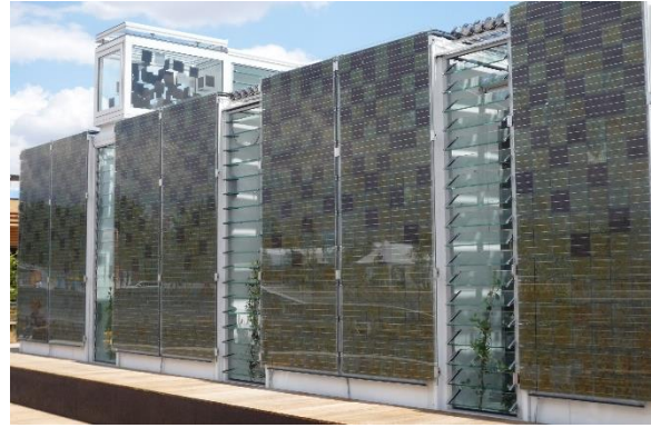
Figure 79: The SDE home+house of the Hochschule für Technik in Stuttgart (HFT) has coloured photovoltaic modules on the façade as its definitive design element Source: University Wuppertal, Karsten Voss
