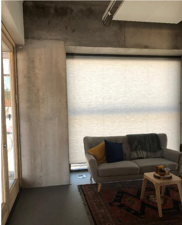
Figure 55: Massive constructions are not common in the SDE context. Because teams only have 10 to 14 days to assemble their houses on the event site and all houses need to be transportable, constructions based on reinforced concrete are not feasible. However, the SDE 2019 focused on existing building renovations and the organizers gave all teams the unique possibility to request a building structure that would be built prior to the arrival of the teams. Only the teams DEF (MOR of the TU Delft) took advantage and requested a concrete structure. This structure is kept visible from the inside. Source: University Wuppertal, Susanne Hendel
