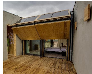
Figure 28: Foldable external sun protection additionally used for solar power generation at the SDE 2014 ROF house. Source: SDE, Flickr, Valeria Anzolin, Jason Flakes [sde flickr doc]
