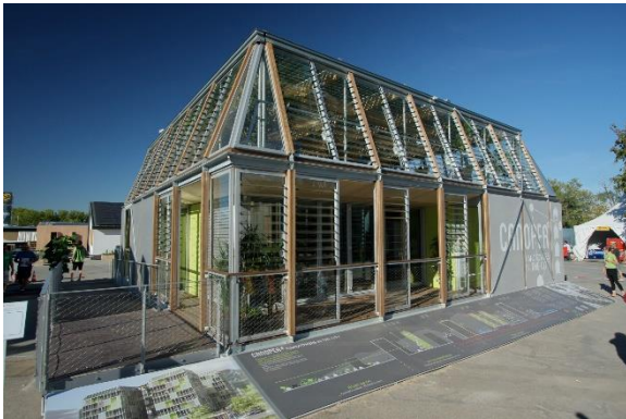
Figure 35: Exterior view of the Canopea house of the French 2012 TRA team. The unit demonstrated the upper floor with an additional buffer zone on top of an urban apartment building. Source: SDE, Flickr [sde flickr doc]
