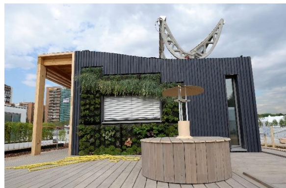
Figure 48: Green façade at the SDE 2010 AMP house. Source: SDE, Flickr [sde flickr doc]
