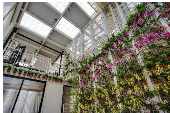
Figure 32: Exterior buffer conservatory at the 2014 UNI house, with advanced functionality. Source: SDE, Flickr, Valeria Anzolin, Jason Flakes [sde flickr doc]
