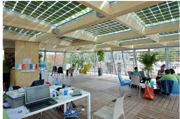
Figure 36: Interior view of the 2012 TRA buffer zone. The roof integrates PV modules for solar power generation. Source: SDE, Flickr [sde flickr doc]
