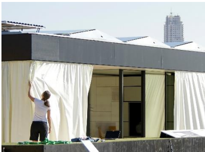
Figure 26: Overhang combine with external curtains at the SDE 2012 RWT house. Source: SDE, Flickr [sde flickr doc]
