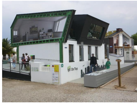
Figure 142: The OTP "On Top" house from SDE 2014. Source: K. Voss, University Wuppertal
