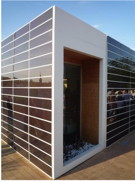
Figure 82: One example of the integrated geometry of solar modules on the facade of the SDE 2010 SML house (CEU). Source: University Wuppertal, Karsten Voss
