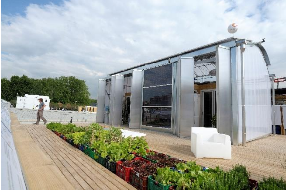
Figure 34: A meeting house for a local district with a translucent façade at the SDE 2010 UPC house. The construction is based on typical greenhouse elements such as multilayer polycarbonate plates. Source: SDE, Flickr [sde flickr doc]
