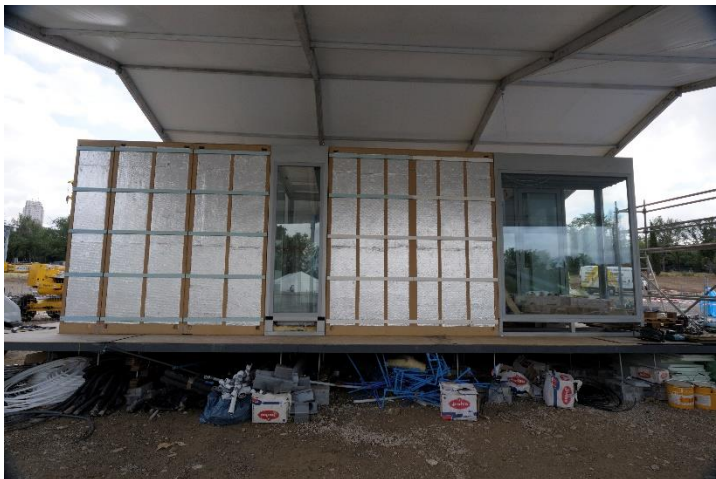
Figure 57: Vacuum insulating panels visible at the 2010 UDS (Solarkit) house during assembly. Source: SDE, Flickr, Javier Alonso Huerta [sde flickr doc]
