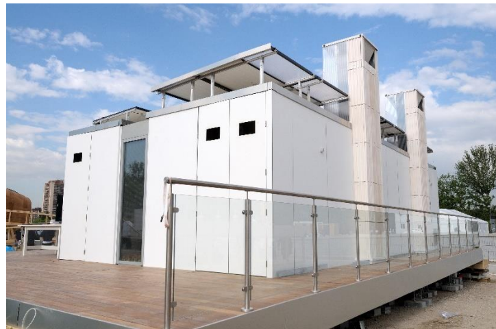
Figure 40: Solar chimney at the SDE 2010 UDS house. Source: SDE, Flickr [sde flickr doc]
