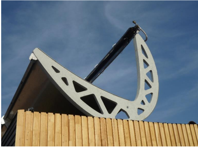
Figure 110: Concentration solar thermal system on the roof of a house at SDE 2010. Source: K. Voss, University Wuppertal
