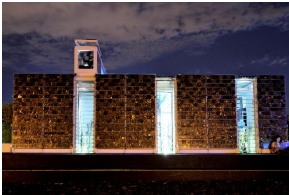
Figure 96: home+ (HFT) at SDE 2010 is a good example of the visible use of crystalline PV modules over a large area. Modules were integrated into the roof and also into the facade of the building, where coloured cells were part of the design. The PV areas together are about twice as large as the floor space. Source: [sde flickr]
