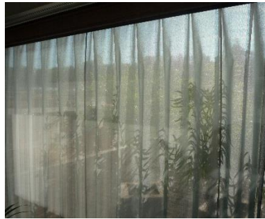
Figure 24: View through an external curtain as a moveable sun protection device presented by the SDE 2010 Wuppertal house (BUW). A transparency of 7% is sufficient for visual contact. Source: University Wuppertal, Karsten Voss
