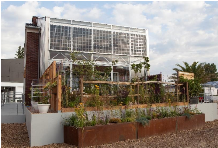
Figure 30: The attached conservatory at the 2014 DEL house with integrated solar systems demonstrates a buffer zone example for building renovation. Source: SDE, Flickr, Valeria Anzolin, Jason Flakes [sde flickr doc]
