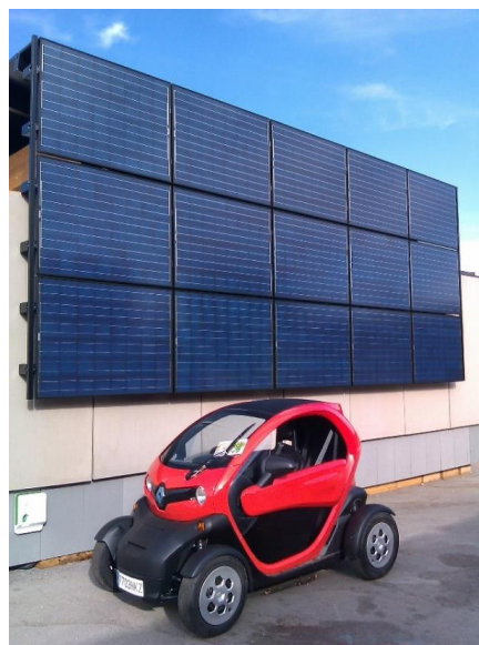
Figure 85: Solar system on a non-dominant substructure extending beyond the roof and over part of the façade of the SDE 2012 Med in Italy house (ROM). Source: University Wuppertal Karsten Voss
