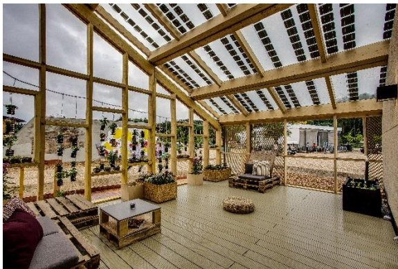
Figure 98: At SDE 2014, installed PV system capacity had already been limited to 5 kW p . One example of the relatively small PV systems at the competition is the DTU 2014 house. Individual modules were integrated into the glass roof of an outer buffer zone. Source: SDE Flickr, by Valeria Anzolin and Jason Flakes [sde flickr]
