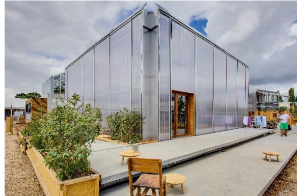
Figure 62: Translucent façade cladding at the SDE 2014 BAR house. Source: SDE, Flickr, Valeria Anzolin, Jason Flakes [sde flickr doc]
