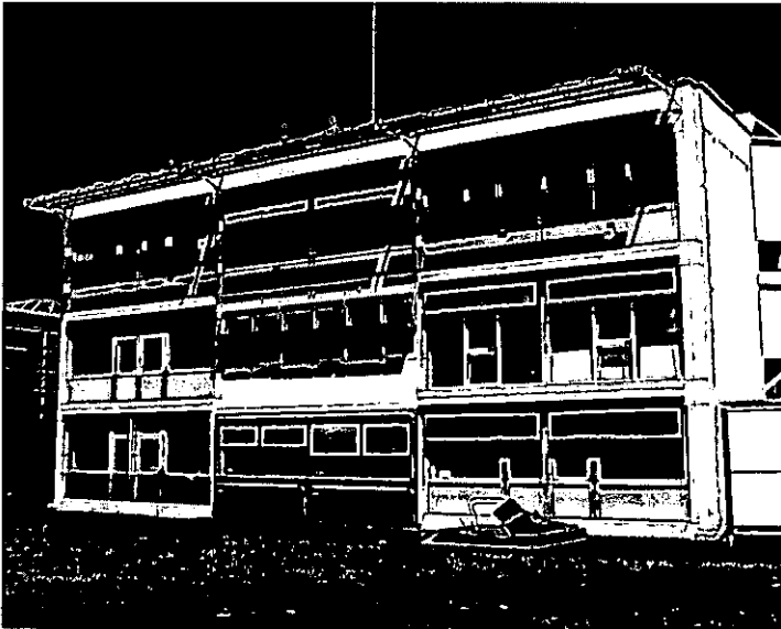
Figure 7.5 Building 4 - 3-storey office building, Switzerland
