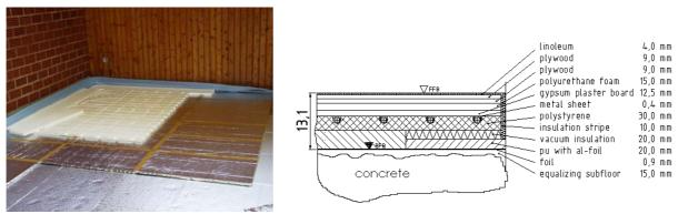
Figure 69: Left: Photograph of the floor during the installation. The shiny VIP are put on the matt aluminium layer of the polyurethane boards. The VIP were connected with tape. White polystyrene plates with grooves for the heating pipes are mounted on top of the VIP. Right: Cross-section of the floor insulated with polystyrene as well as with VIP
