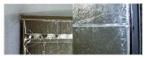
Figure 57: Gaps and edges of VIP in the elements left: va-Q-tec AG VIP right: WACKER CHEMIE VIP
