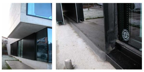
Figure 34: Façade detail with sliding elements in rest position in front of VIP wall elements
