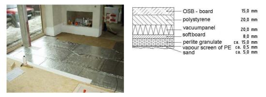
Figure 67: Left: Photo taken during renovation. The OSB can be seen in the foreground, the VIP in the centre and the softboard in the background. (foto: may.schurr.architekten, Bad Wörishofen)
