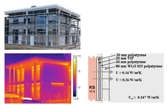
Figure 62: Left: View of the house from the south-west; several polystyrene-encased VIP are already mounted. Thermographic image taken after the second layer of insulation was mounted.
