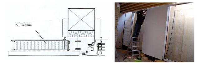
Figure 4: Vacuum insulation panels in the form of stainless steel cases used as outside wall elements on single-family terrace houses in Binningen / Switzerland Left: Horizontal section through the construction Right: Installation of the VIP (Architect: Ecinor Postolozzi, Posel (Switzerland; Eccade system; Höring AG, Switzerland)
