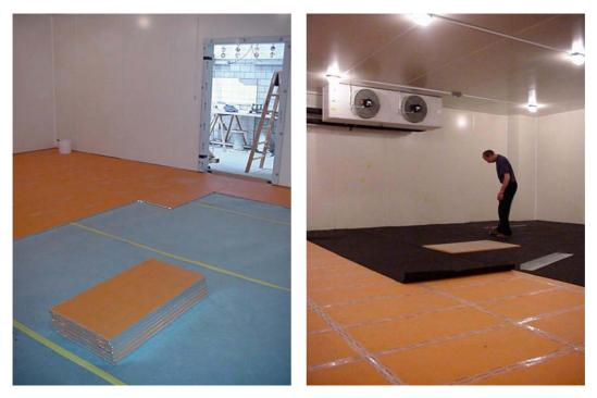
Figure 30: Building site of the floor insulation
