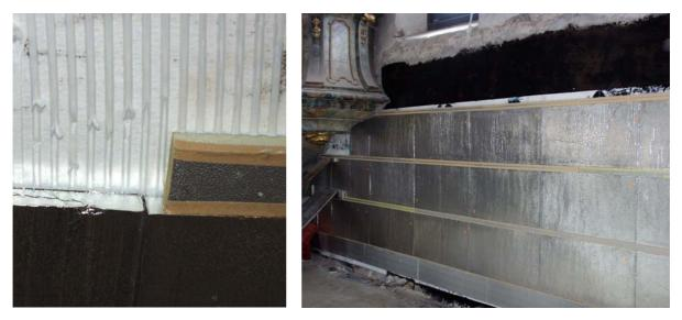
Figure 52: Left: Installation of the VIP with dispersion based mortar onto the polysterene boards. The horizontal strips of polyurethane can be seen as well as the vertical strips of dispersion based mortar.
