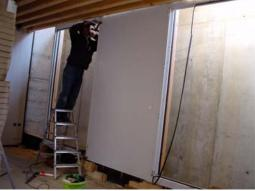
Figure 38: Left: Horizontal section through the construction Right: Installation of the VIP
