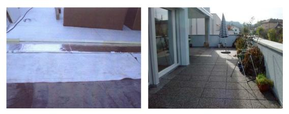
Figure 29: Building site – finished terrace: VIP is already well protected during installation.
