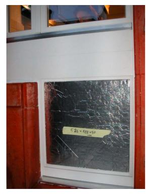
Figure 36: Window element with tight-fitting VIP
