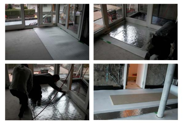
Figure 22: Worksteps in building up the floor
