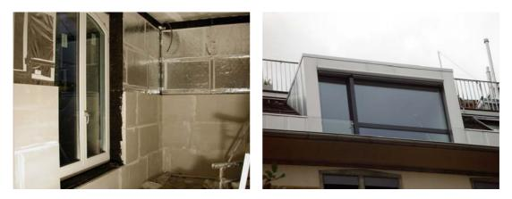
Figure 25: Left: Interior VIP insulation with gypsum board walling in front Right: Finished dormer window
