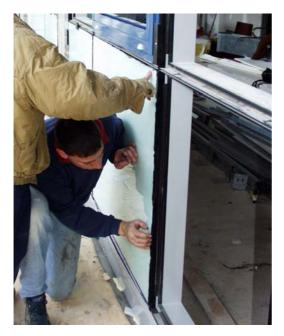
Figure 56: Photograph of the vacuum-insulated façade elements being installed
