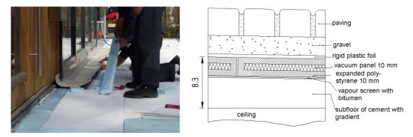
Figure 66: Left:Installing the polystyrene-encased VIP. The border between the floor and the house was filled with pieces of polystyrene. (foto: may.schurr.architekten, Bad Wörishofen) Right: Insulation design
