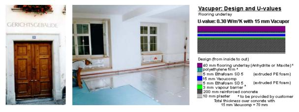
Figure 68: Left: Entrance area of the historic court house in Schaffhausen / Switzerland. The doors inside the building originate from the 17th century as well and had to be retained. Middle: Mounting the vacuum panels according to an assembly plan. VIP with irregular, slanted sides had to be specially supplied for the edges of the room. All the VIP were numbered according to the plan.
