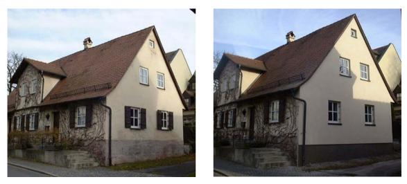
Figure 39: Photograph of the house before and after the gable was insulated
