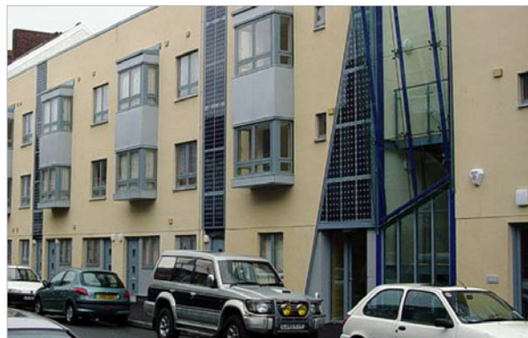
Town houses (Llanelli, Wales)
