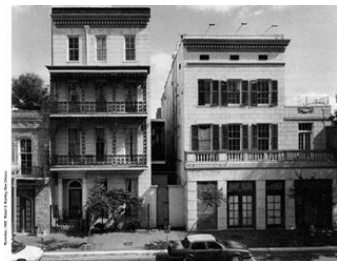
Year 1993 - Both buildings endured vigorously into the 1990s, gaining character and individuality with every decade. Shortly after they were built, both acquired cast-iron balconies on the front and side. Number 822 (left) kept its, but 826 (right) moved on to other additions in three directions—an attic-story upward, an annex to the side and expansion of the ground floor out to the sidewalk. Meanwhile 822 added a full story on top. By 1936, both facades had been coated with stucco, scored to look like stone masonry. A 1970s photo of 826 showed a barbershop in the ground floor. Since that photo, the building acquired shutters, lights on top, a metal railing for the annex deck, and French doors on the ground floor
