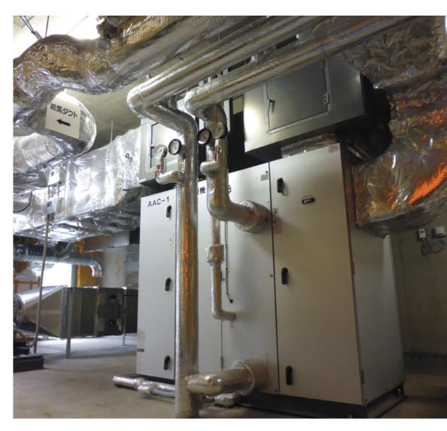
An experimental facility for HVAC systems, showing an air handling unit undergoing testing. Source: Building Research Institute, Japan
