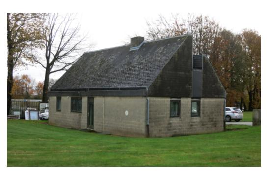
The IDEE house at Limelette, Belgium, a full-scale experimental building that has been used as a test case to develop and evaluate methodologies to characterise the overall heat loss coefficient based on static and dynamic measurement campaigns. Source: BBRI, Belgium
