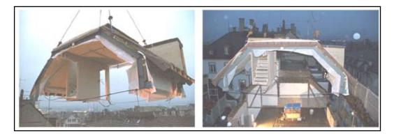
New roof elements are lifted onto the building. The new roof is completed within hours.
