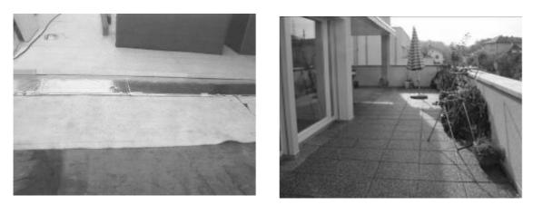
Figure 7: Terrace insulation - during installation and the finished terrace.
